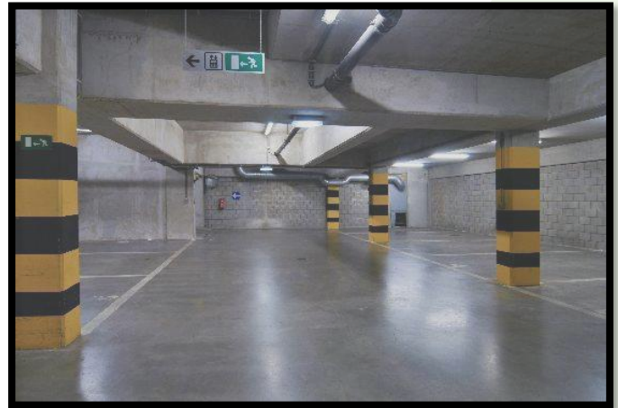
Figure 2 Underground Car Park - Apartment Building
